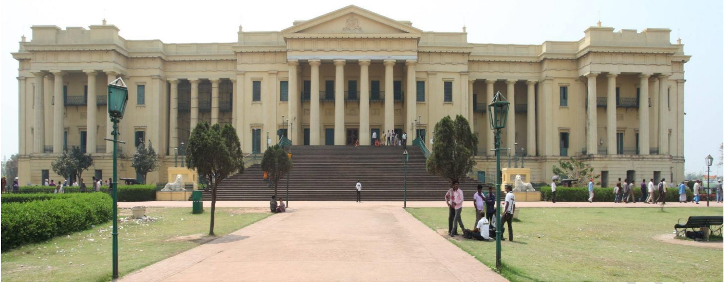
Hazarduari Palace, Murshidabad
